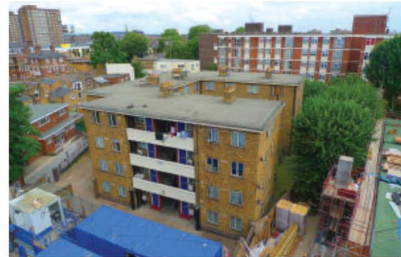
Access decks and London stock brickwork have been replaced by ...
