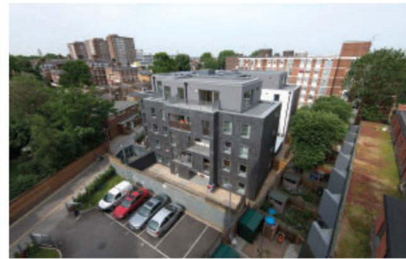
... new balconies, Corian brick slips and a new storey
